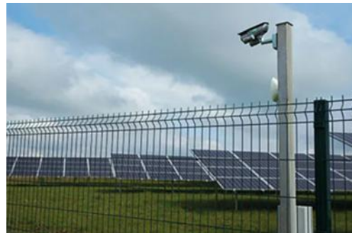
Reality: LPS 1175 issue 8.1:D10 fencing
